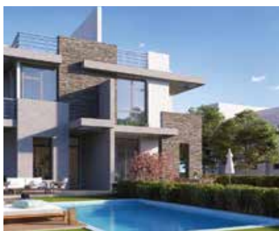
The Thousand Villas Project
