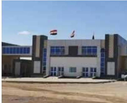
EAST OWAINAT Project
